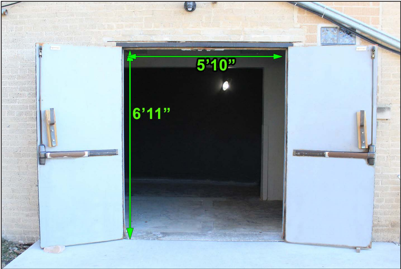
SOUTHWEST DOCK DOOR 1
