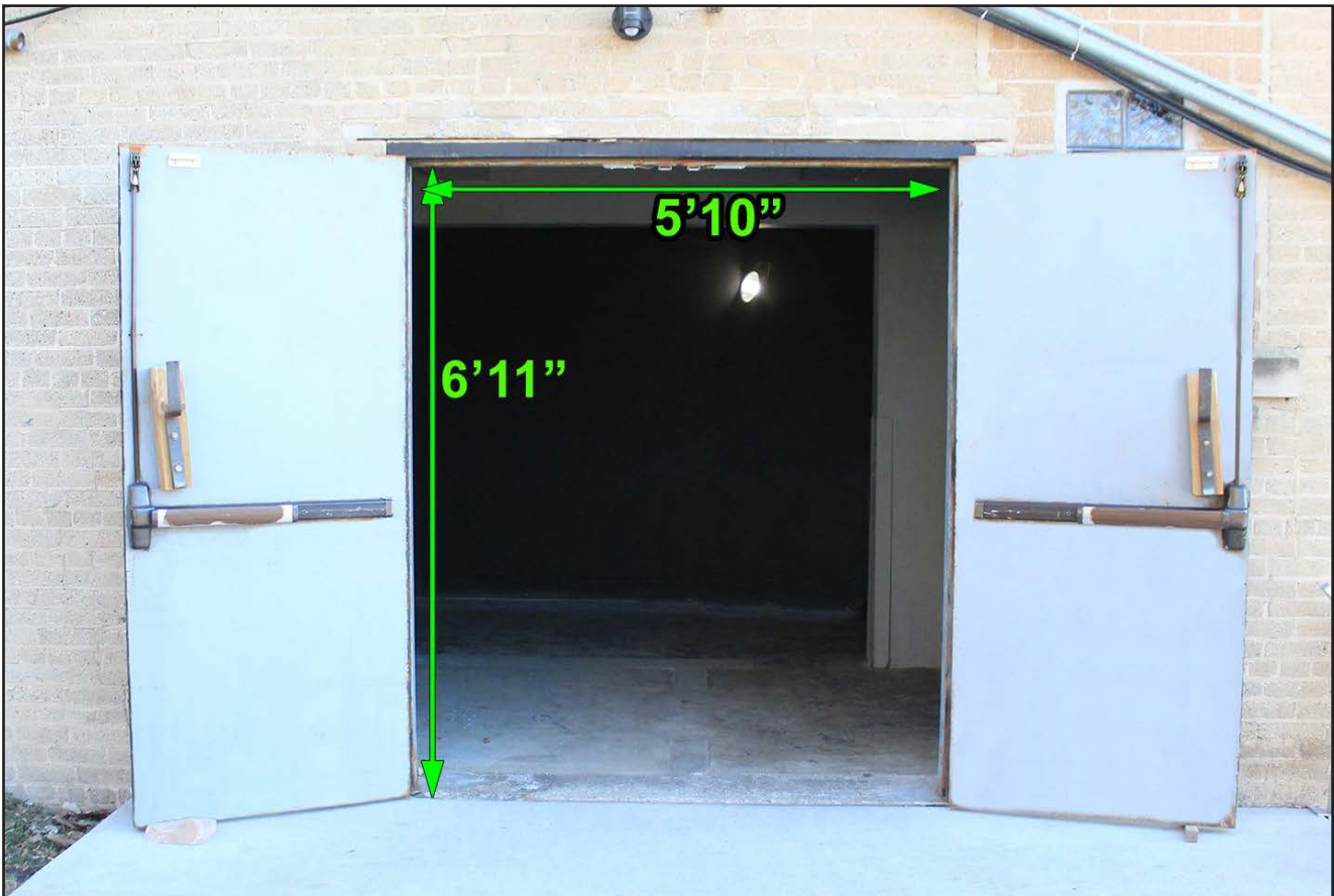
SOUTHWEST DOCK DOOR 1
